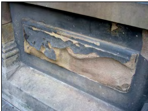
Eroding stonework in The Strand.
