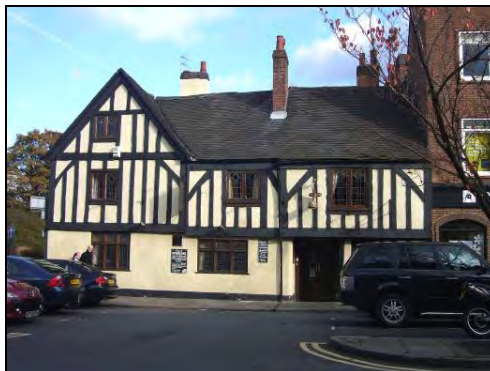
22 Iron Gate (left) has the characteristic twin gables and jetty of a 16 th timber framed house; The Dolphin's timber frame (right) is still exposed (though much restored).
