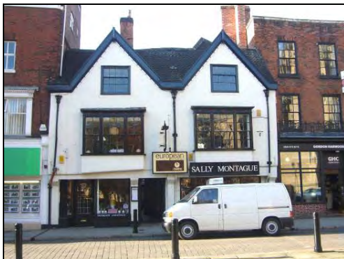
22 Iron Gate (left) has the characteristic twin gables and jetty of a 16 th timber framed house; The Dolphin's timber frame (right) is still exposed (though much restored).
